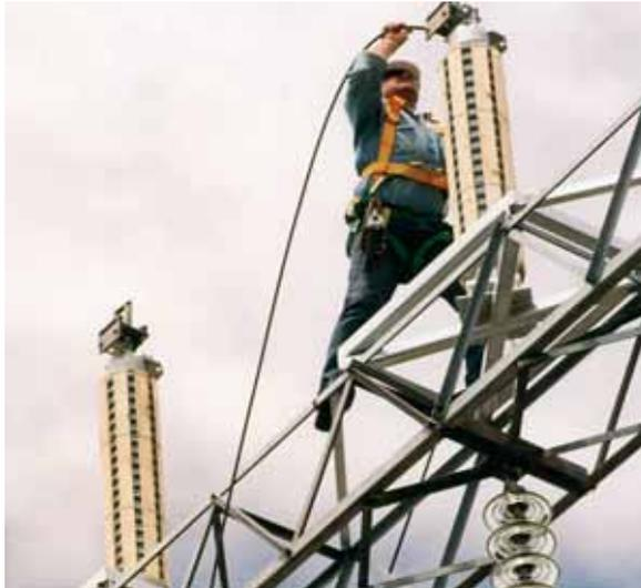
TRANSMISSION LINE COMPLIANCE: Post insulators were attached to a tower on the Tungatinalh–Waddamana 110 kV transmission line by a crew from Aurora energy. The objective of the work was to raise the heights of conductors to meet contemporary conductor-to-ground clearances.
