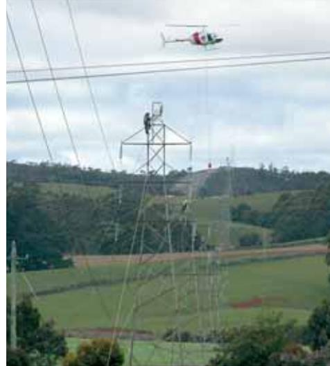
*OPTICAL FIBRE GROUND WIRE An OPGW being installed on the transmission line between Burnie and Smithton substations. (Photo courtesy of Electrix Pty Ltd)*
