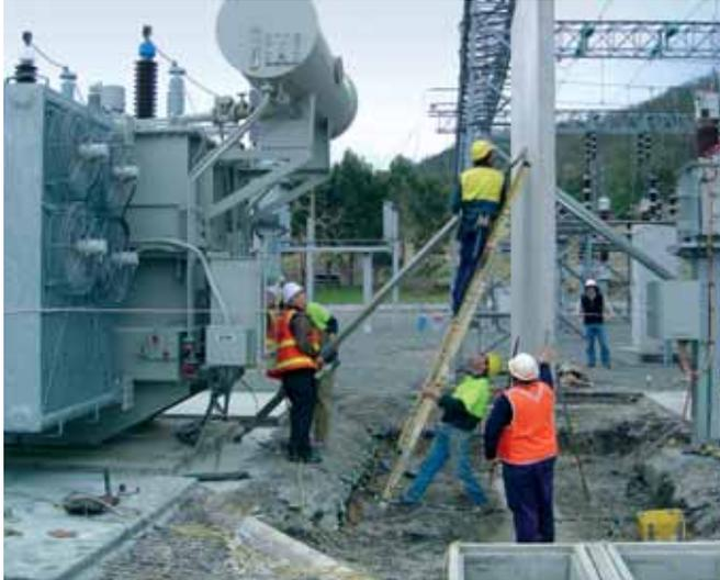
*OIL CONTAINMENT: A blast wall was installed at Knights Road Substation, Huonville, as part of Transend's program to build contemporary oil containment facilities at all its substations.*
