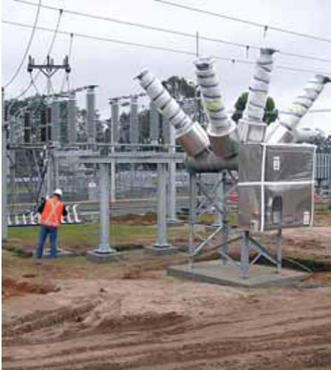
*NORTH-EAST REDEVELOPMENT: A new 110 kV circuit breaker is being installed at Scottsdale Substation as part of the substation redevelopments in north-east Tasmania. (Photo courtesy of John Copas, Enerserve)*
