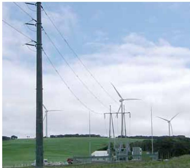
*WIND FARM CONNECTION: Hydro Tasmania’s Woolnorth wind farm is connected to the transmission system by a new 110 kV line to Smithton Substation.*
