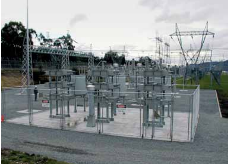
CAPACITOR BANK: A capacitor bank was installed at Transend's Chapel Street Substation during 2003-04.
