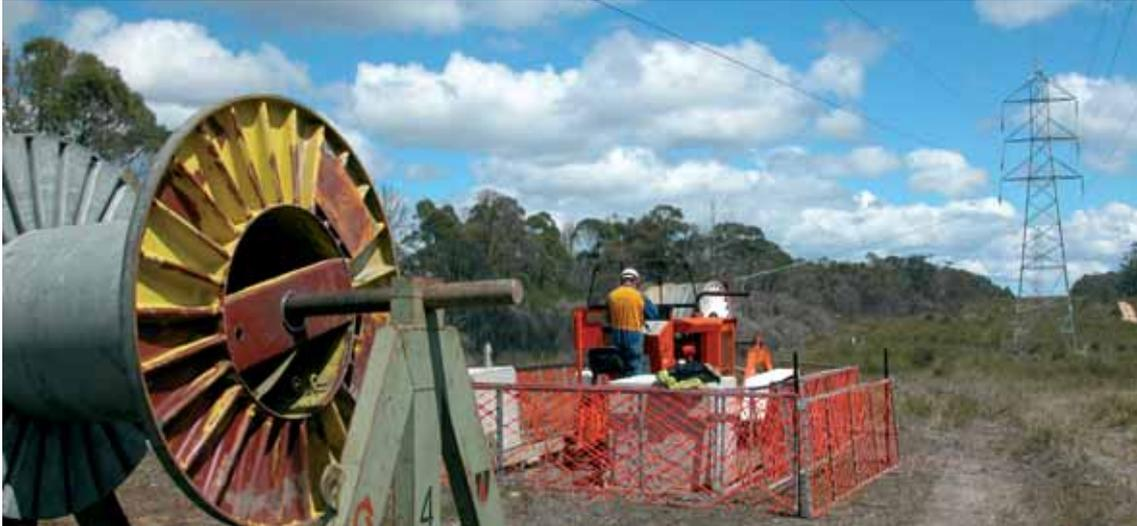
SECOND CIRCUIT: The second circuit being strung on the Burnie-Smithton transmission line as part of the redevelopment of the transmission system in the Circular Head area (Photo courtesy of Electrix Pty Ltd)
