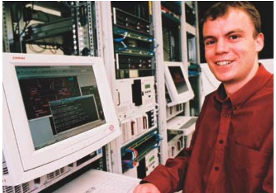
NETWORK CONTROL: Ian Stewart, an engineer with Open Systems International Australia, has been involved in building Transend's network operation and control system—the hardware and software that will control Tasmania's transmission network.
